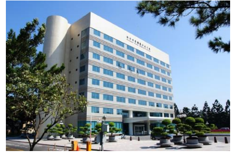
Monitor offices & buildings
