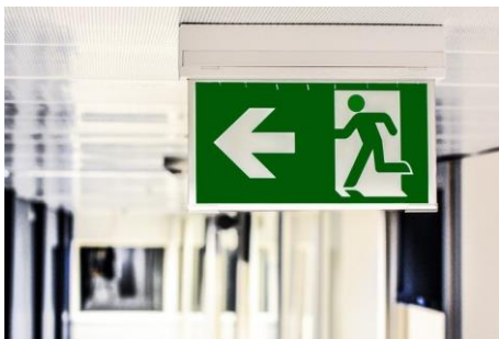
Protect emergency door
