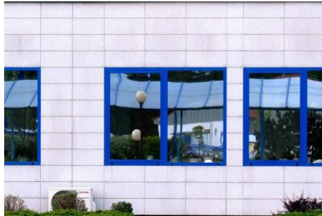
Guard office windows
