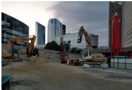
Guard construction sites
